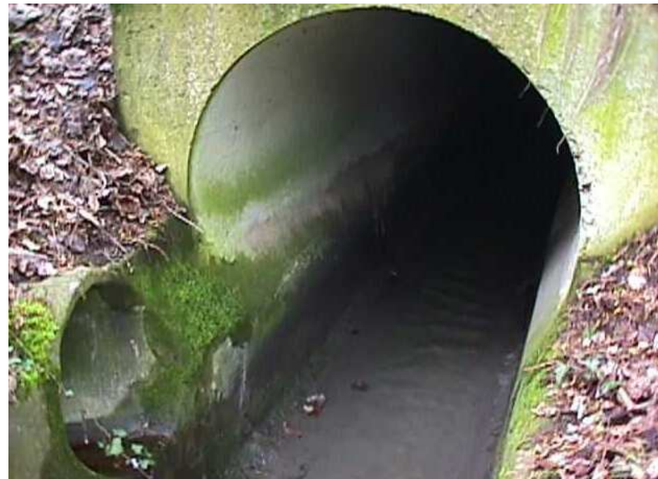
Pt 171 is located in this pipe
