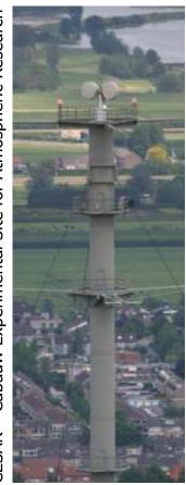
IDRA is mounted on top of the 213 m high meteorological tower.
